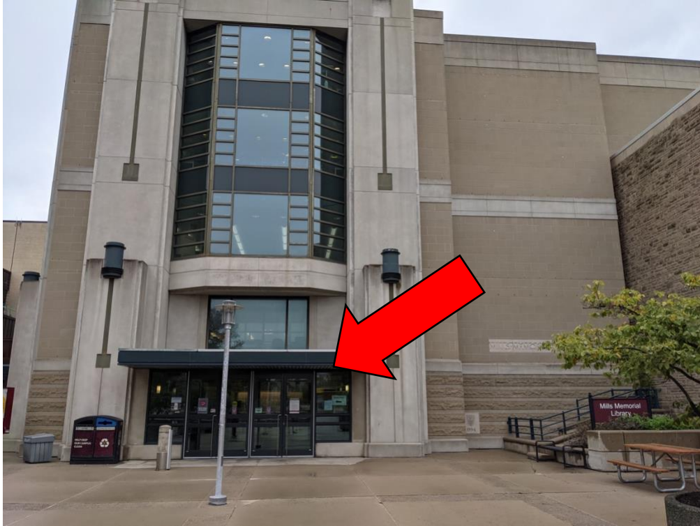
Entering the building (west side).
